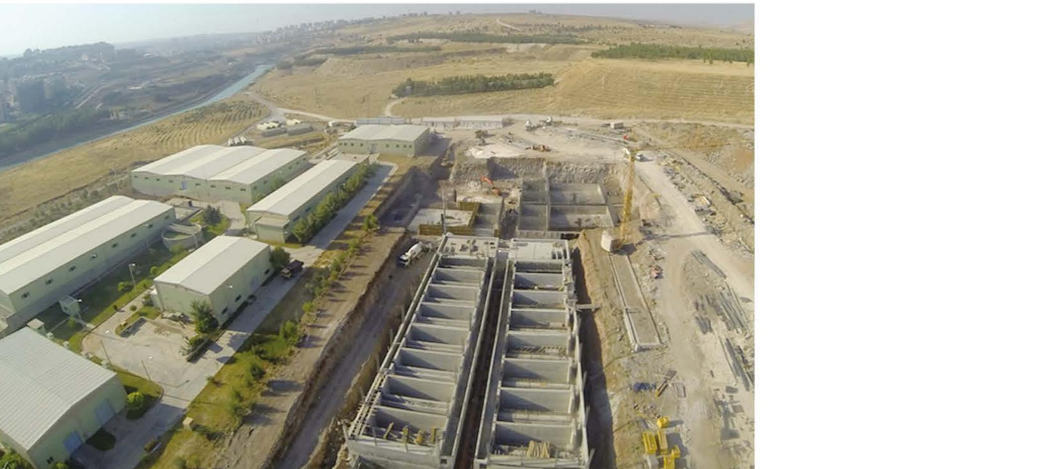
While the capacity of the existing drinking water treatment plant was 270 thousand cubic meters per day, with the completion of the second stage, the capacity increased to 540 thousand cubic meters per day.
