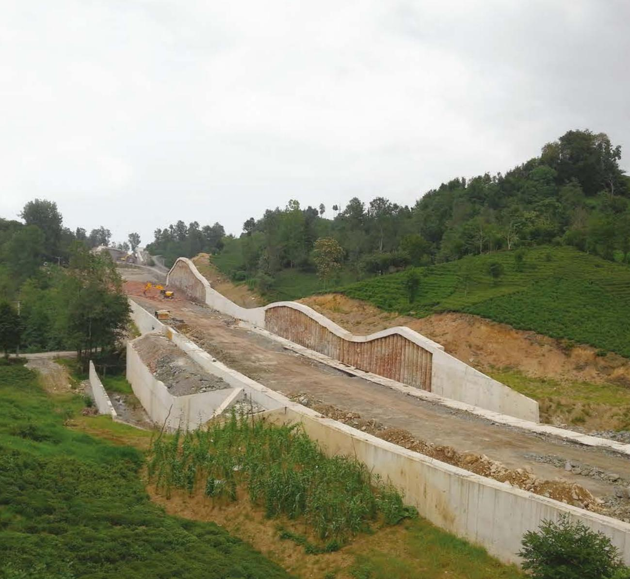
455.000 m<sup>3</sup> excavation works, 415.000 m<sup>3</sup> backfilling works, 3,800 mt curbstone works, 17,716 m<sup>3</sup> RC culverts works, 15,000 m<sup>3</sup> RC wall works, 40,000 mt piling works, 10,000 tones subbase works, 25,000 m<sup>2</sup> bituminous asphalt works, 4,383 m<sup>3</sup> RC bridge works.
