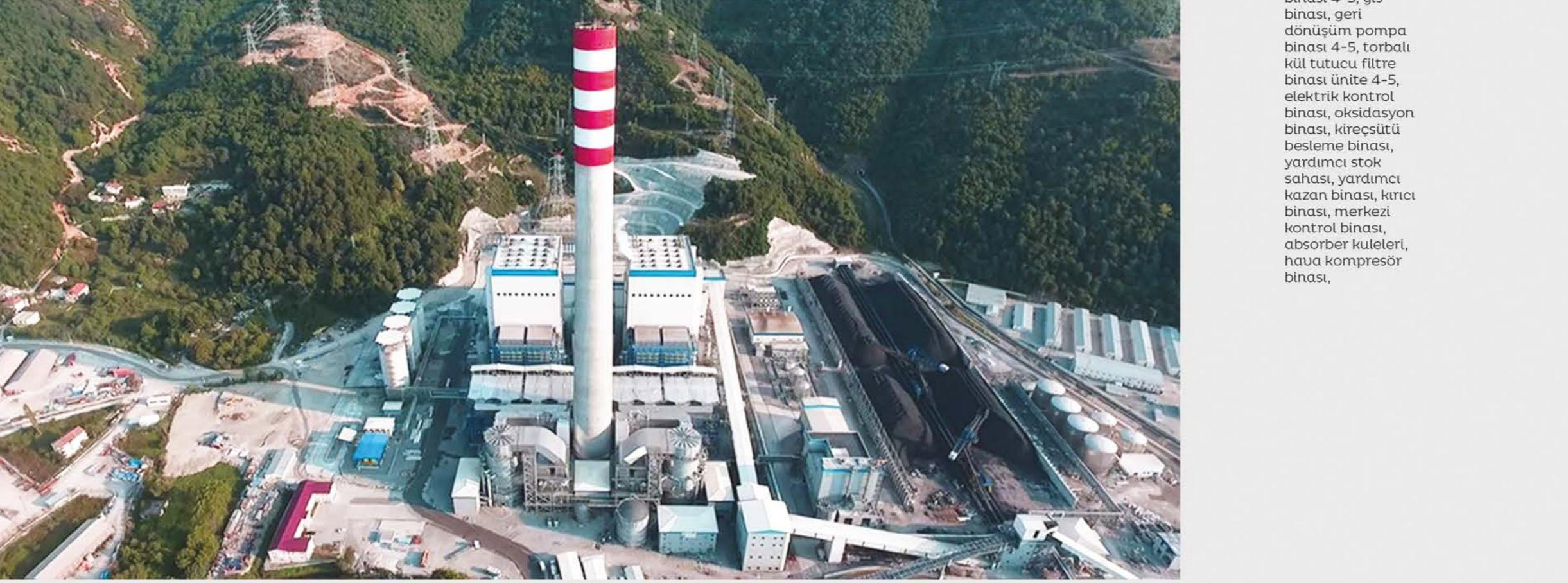
The structures in the project are as follows: turbine building 4-5, boiler building 4-5, gis building, recycling pump building 4-5, ash collector filter building unit 4-5, electric control building, oxidation building, limestone feeding building, auxiliary stock ammonia storage area, wastewater treatment plant, demineralized water tanks, fire pump building, warehouse building, auxiliary boiler building,
